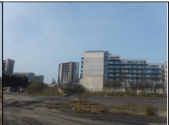
Figure 6.21: View looking west southwest. Most of the existing development in the area around the site consists of 8 storey mixed use blocks. In the background is the shell of a partly completed 14 storey building.
