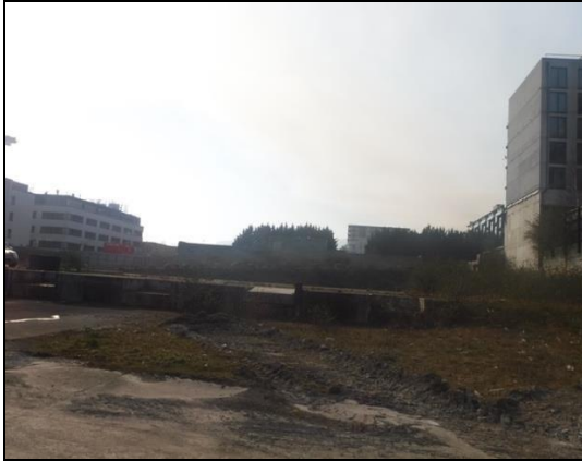
Figure 6.18: View looking south west. The subject site predominantly consists of a hard landscaped brownfield site bound by hoarding.
