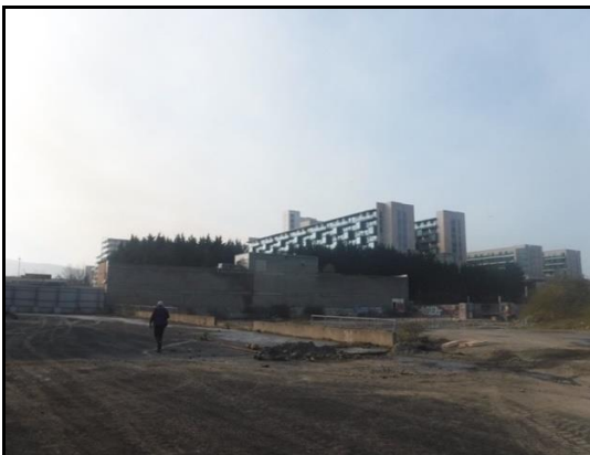
Figure 6.20: View looking south west. Only one structure remains at the south end of the site it is a two storey over basement structure and of late 20 th century concrete block construction. It is of no architectural merit.
