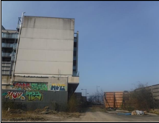
Figure 6.22: View looking directly west towards an existing mixed use block.
