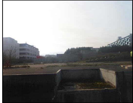
Figure 6.19: View looking south west. The lands to the south predominantly consist of 3-8 storey mixed use office and residential development and low rise industrial estates.
